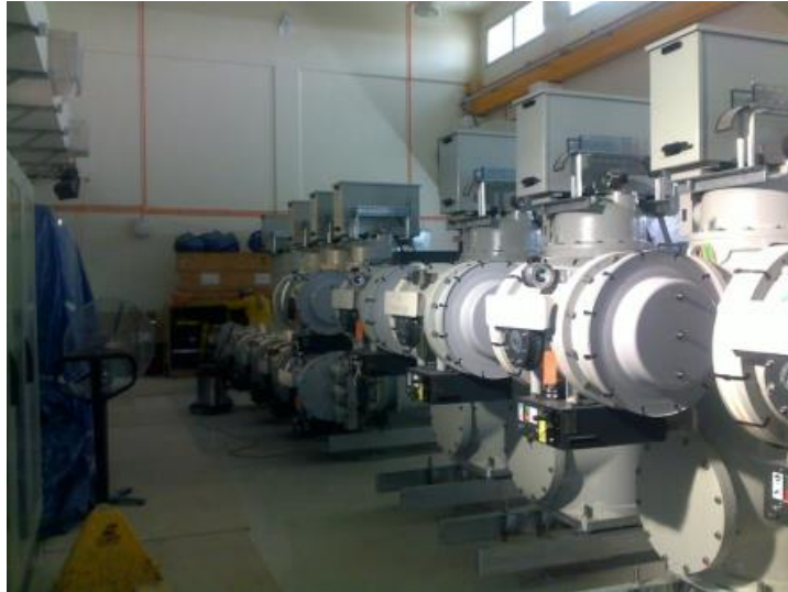
Figure 4. View of a typical floor inside a GIS building
